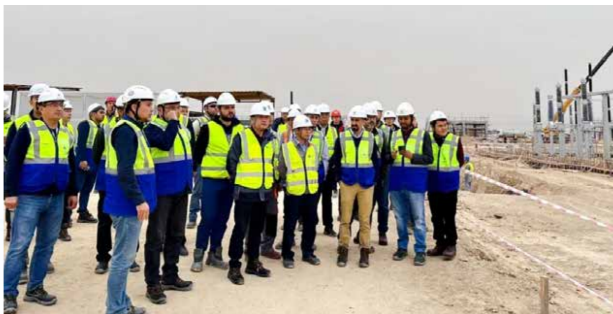
General Manager Fang Yanshui Inspecting the Safety Production Work at the 500MW Sherabad Solar Power Plant in Uzbekistan
